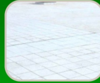
COOLING LIME TILES AT TERRACE
